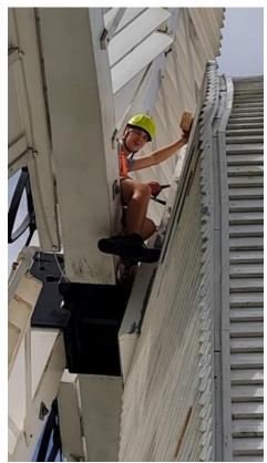
progress was made in the sunny weather until the end of June, but July and August were very wet and windy and completion was delayed until the sun returned in September. Working on the front of the mill is complicated by the sweeps, though standing on the stocks – the large timbers at the centre of the sweeps – does enable the top of the front to be reached.
