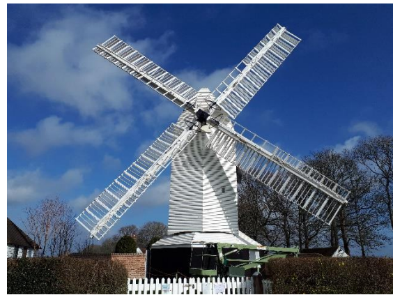
Oldland Mill with Windboards removed for repair and restoration.
