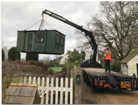
Removal of the old Portacabin
