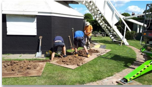
Lightning conductor groundwork
