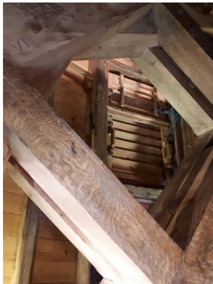
View of the repaired and refurbished Storm Hatch
