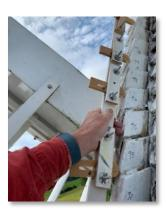
Strakes high on the mill had to be laminated to match the beautiful (but complex) curve of the front of the mill, here measured with a 5-point gauge
