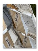
Every single weatherboard needed its own wedge, to provide a level surface for the flashings. Every wedge needed to be individually measured and cut.
