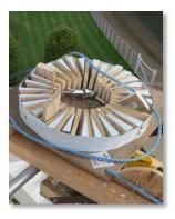
Special 'carousels' were needed to paint and transport the wedges, each individually numbered ready for installation
