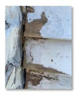
Water penetration was the problem, where the original flashings had failed at the junction of the front and side weatherboards.
